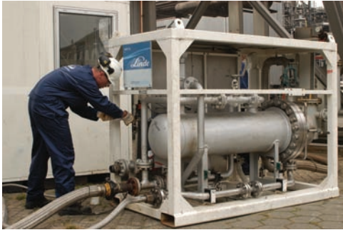
Steam vaporizer capacity 15,000 m 3 /h Nitrogen
